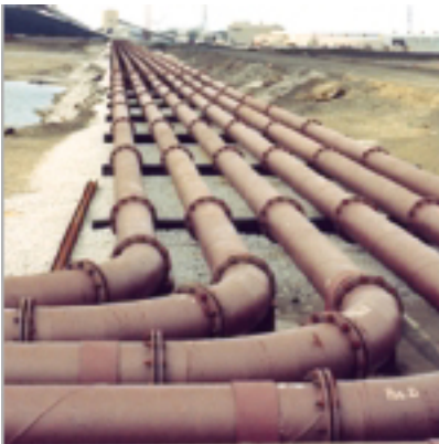
Left: With life times of more than 30 years, ABRESIST pipelines have been used for the hydraulic conveying of ash on all continents. This plant in the U.S. has over 10,000 meters of 294 mm ID pipe in service.
