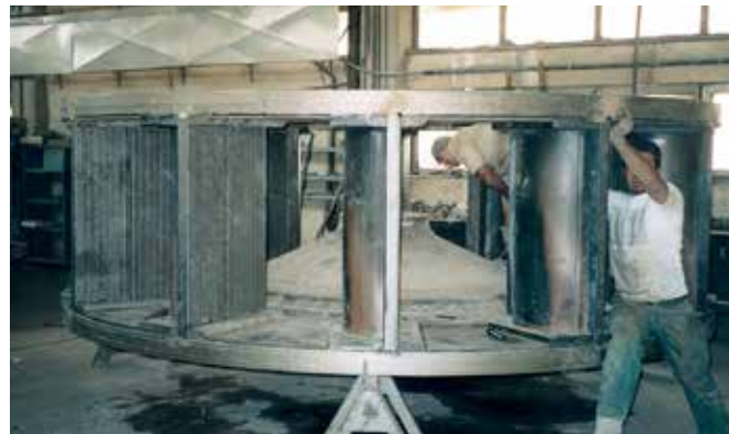
Impact coal pulverizers operate in lignite fired power plants; the impact plates are made of KALMETALL W100.
