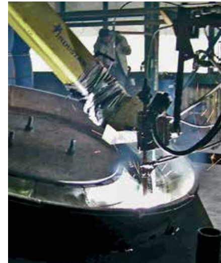
Rebuilding a grinding table with KALMETALL W100.
