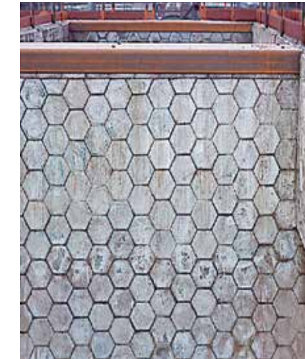
Extended service life of plant components
