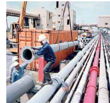
Installation of wet ash pipes in Malaysia (350 mm diameter).
