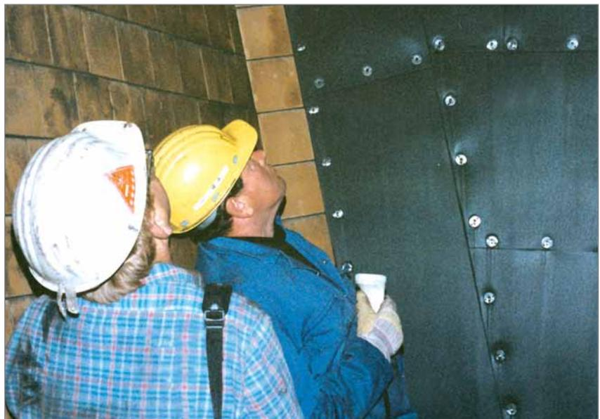
Lining combination in a large fine coal bunker: The surfaces subject to different wear have been protected with due regard to the stress to which they are exposed, here e.g. with KALCERAM and KALEN.
