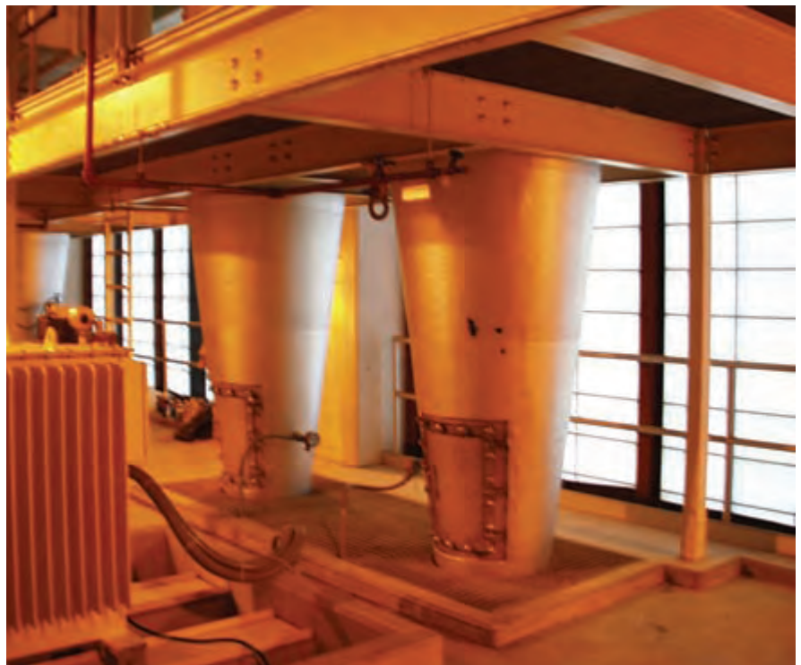
Two cyclones remove airborne dust particles from a dryer's exhaust air before the air is dispersed into the atmosphere.
