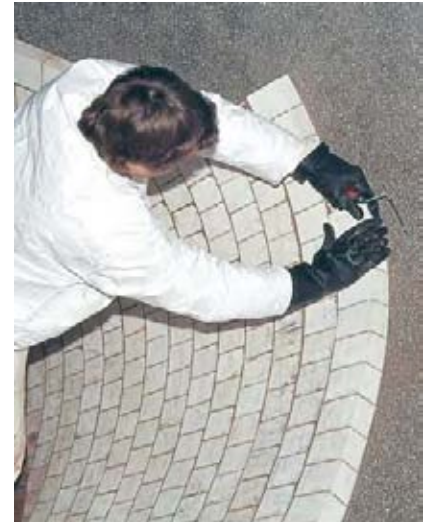
Kalenborn Service solves wear problems on site
