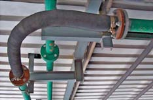
KALFLEX pipe bends in practical operation; here shown as flexible connection between rigid connection points
