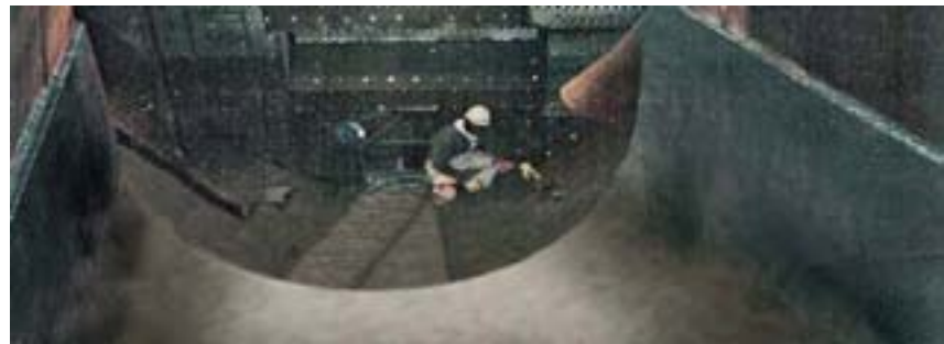
KALCRET hard compound has stood the test as lining material in components of slag granulating systems. Depending on their specific geometry the plant components can be lined within a minimum of time by trowelling or by the spraying technique.
