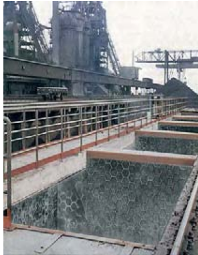
Extended service life of plant components
