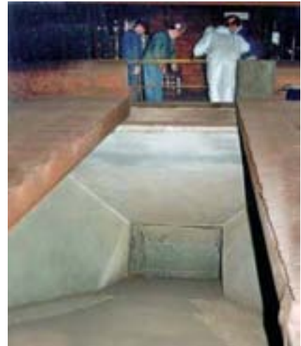
Quick installation of abrasion resistant lining for wind boxes, i.e. sprayed-on KALCRET-BNS hard compound
