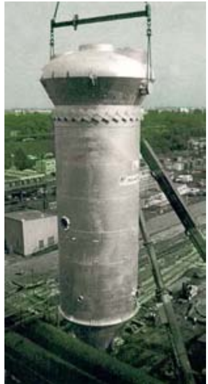
Dust collection cyclones for blast furnaces are effectively protected with KALCOR zirconium corundum
