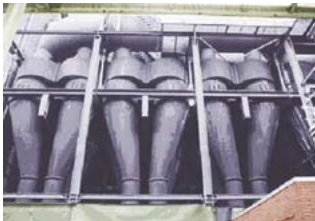
Dust collection cyclones for blast furnaces are effectively protected with KALCOR zirconium corundum
