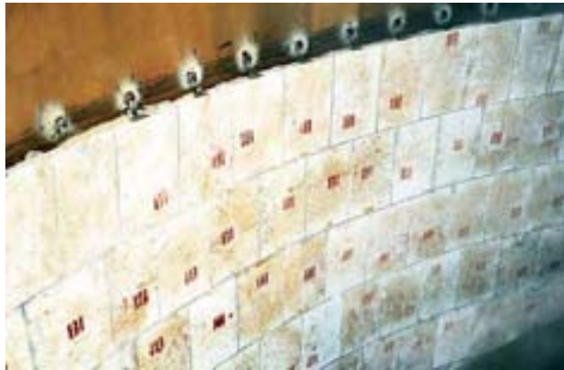
Short lining times for a whirler thanks to sprayed-on KALCRET-BTS hard compound; the high application rate is 5 m 2 /h
