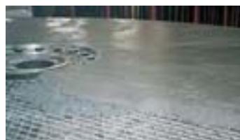
Lining the separator used for cement grinding with KALCRET-BNX, up to 3,200 mm Ø
