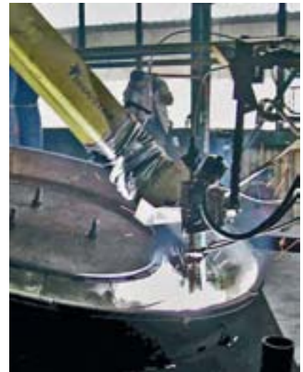
Kalenborn Service solves wear problems on site
