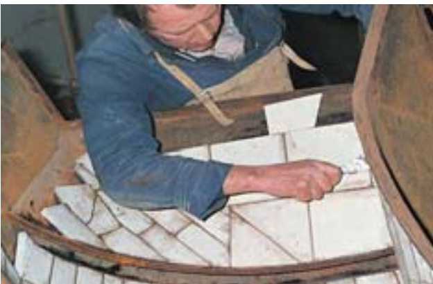
KALCERAM hard ceramics lining for a chute of a cement bag loading system
