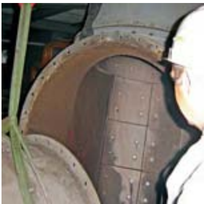
Discharge chute lined with KALMETALL-C, 25 mm thick; fastened with countersunk screws
