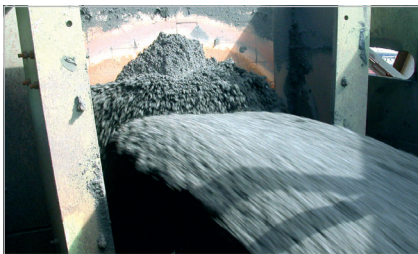
KALIMPACT lining fitted to a bunker in a loading and unloading plant
