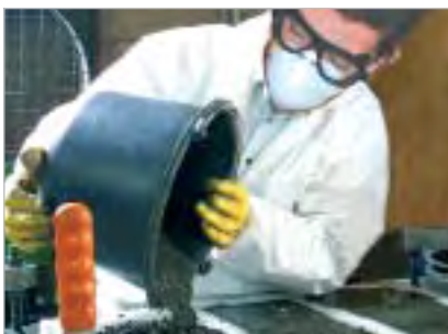
3. Carefully fill formwork
