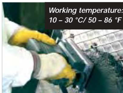
2. Generously apply compound and compact it
