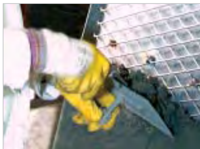
1. Prepare compound to be trowelled as instructed
