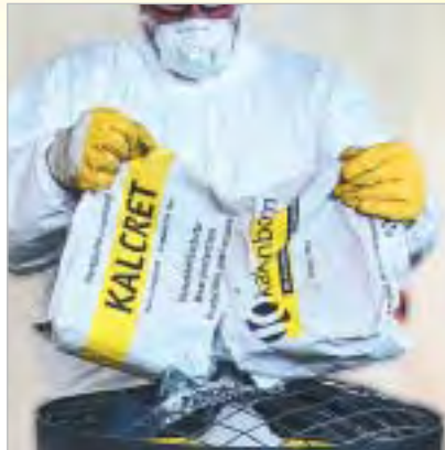
1. Empty the bag of KALCRET hard compound in the mixer
