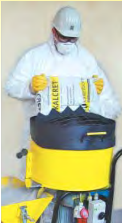
Working with KALCRET spraying system
