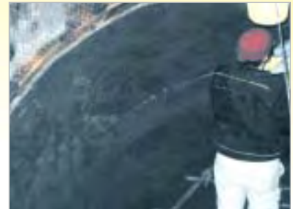
Raw meal duct in a cement plant
