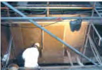
Lining of the impact wall of a coke loading bay
